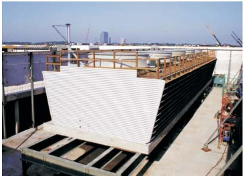
**Series O10** and **Series O15** cooling tower are field constructed, splash fill, crossflow cooling towers, designed to serve all normal cooling water systems as well as those “dirty water” systems which would place the long term operation of a film-fill tower in jeopardy. The principle reason for this reputation is our recognition that each component of a cooling tower must perform at its peak --- and all work compatibly toward overall efficiency.
